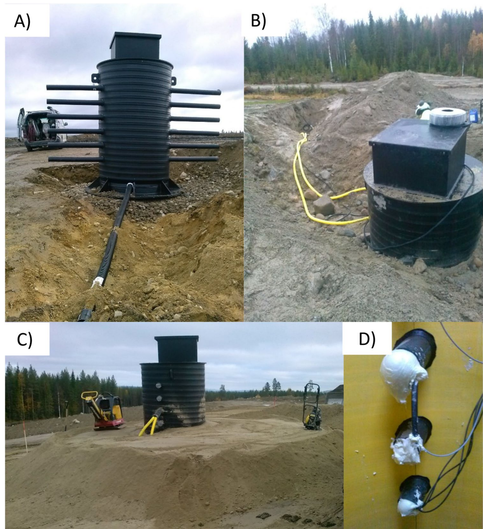
Fig. 3 A A picture of one of the monitoring wells installed in the dry cover. B One of the pits and the cables from the instruments that led to the monitoring wells. C The hand-compacted sealing layer closest to the wells. D The connection from the probes to the wells were insulated first with local material and then with foam insulation and silicon to keep them sealed from atmospheric influence
